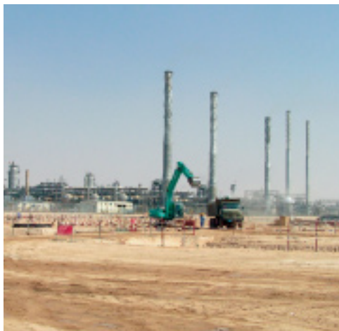
Tihama (under construction), Saudi Arabia
