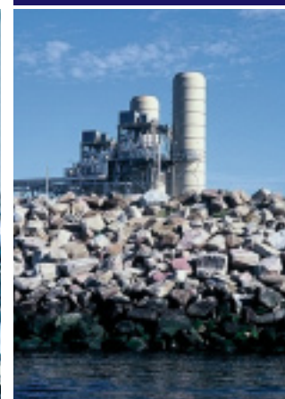
Pelican Point, Australia
